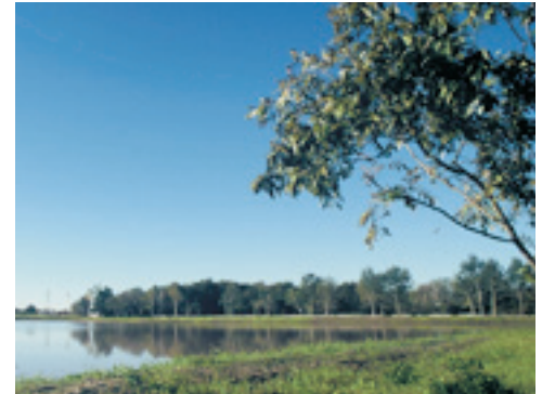
The second phase of construction on the Willow Waterhole Stormwater Detention Basin is on the list of projects approved for funding in 2005.
